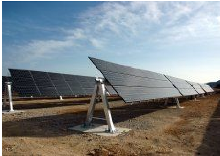
Figure 1.8: Horizontal Axle Mount
